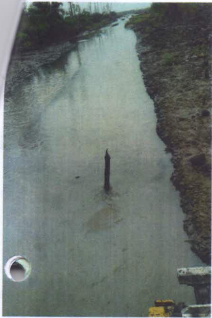
Spill point before excavation.
