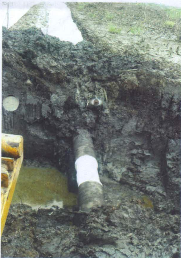
Repairs of the spill point after rapping.
