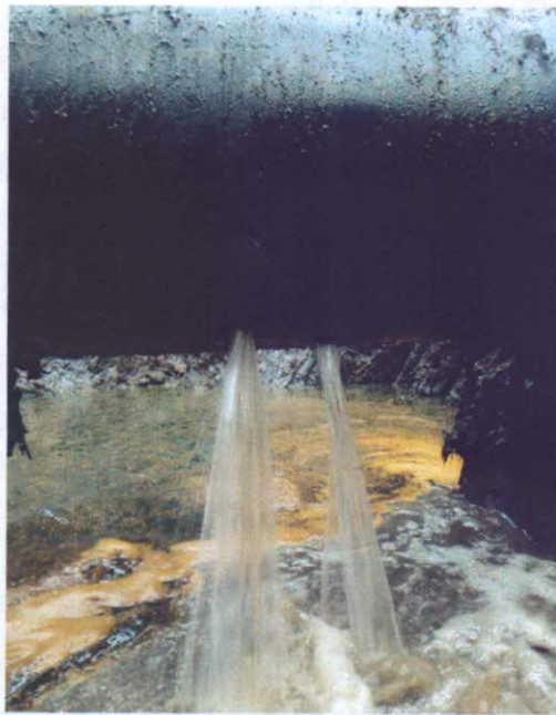
Spill point after excavation.
